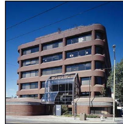
260 Townsend St., San Francisco (1986, renovated in 2002)
